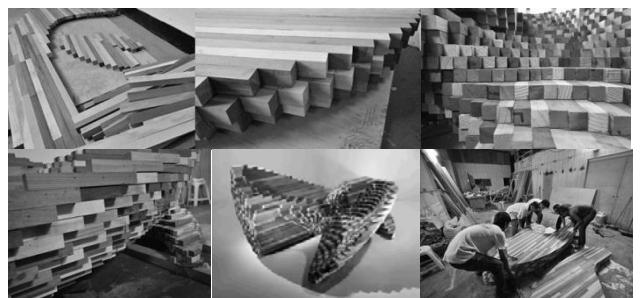
Figure 11 – The process of construction
